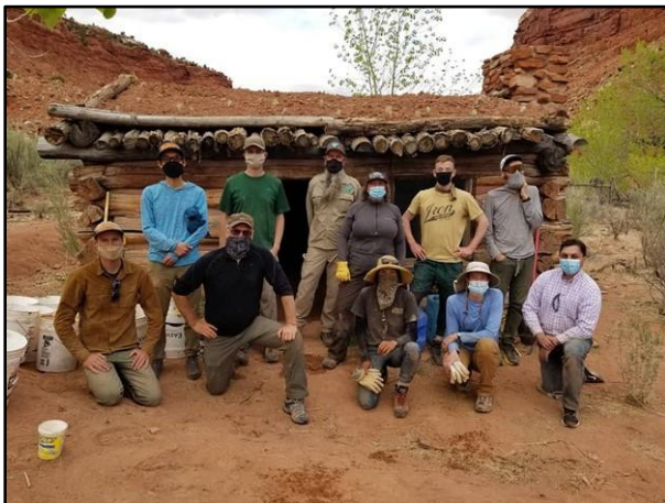
Figure 8: Volunteer group at newly completed Watson Cabin stabilization, GSENM.
