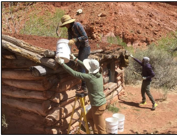
Figure 7: Volunteers working to stabilize Watson Cabin in GSENM.
