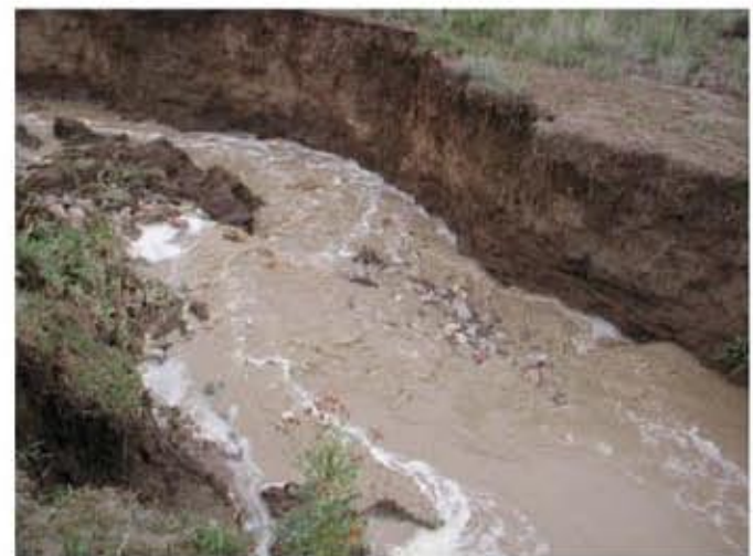
NATURAL DRAINAGE SIDE-CUTTING AS A RESULT OF STORM RUNOFF.
