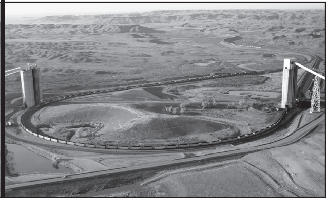
Loadout Facilities in Porcupine Creek Valley North Antelope Rochelle Mine, Wyoming
