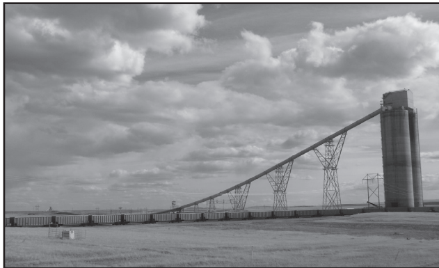
West Loadout Facilities Black Thunder Mine, Wyoming
