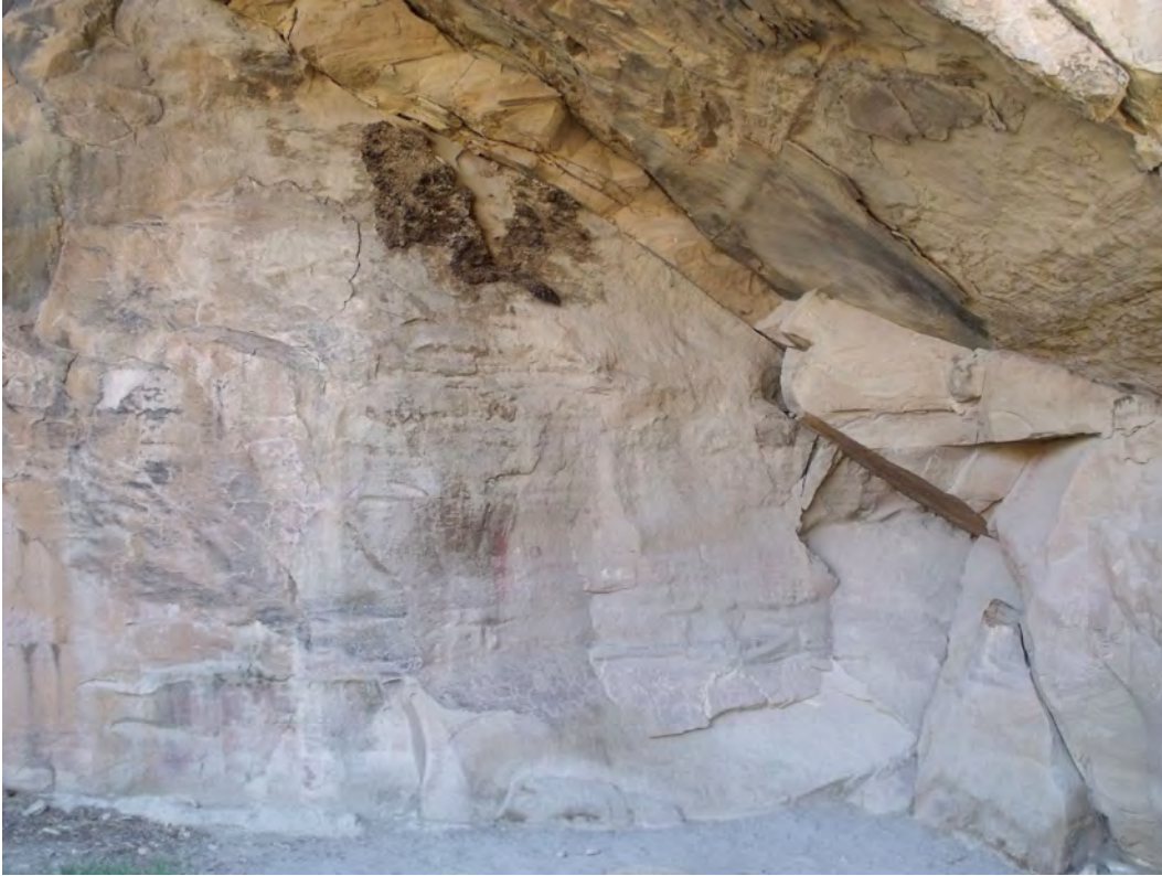
Figure 5. Pack rat urine, dust, graffiti and attempted removal of element at First Site (42Cb1279).
