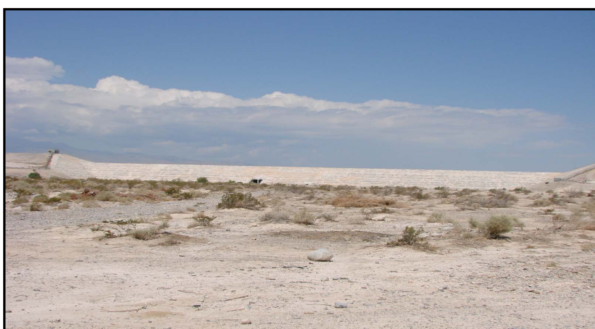
Detention Basin for flood control within the ULVW – CTA.
