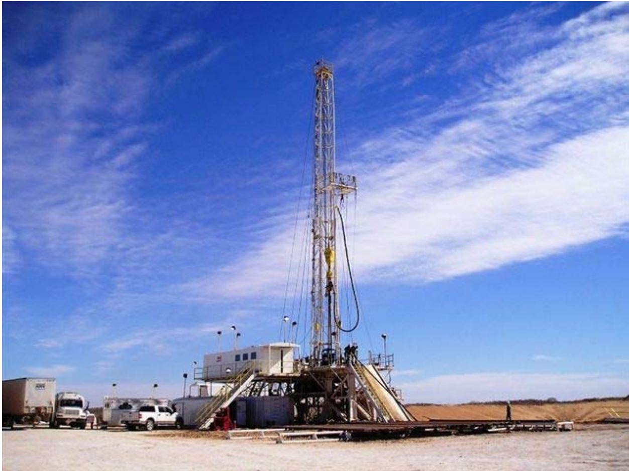
Figure 2-3 Photo Depicting a Typical Drill Rig
