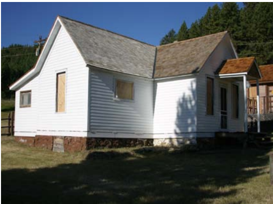
The Zortman Guard Station; after renovations
