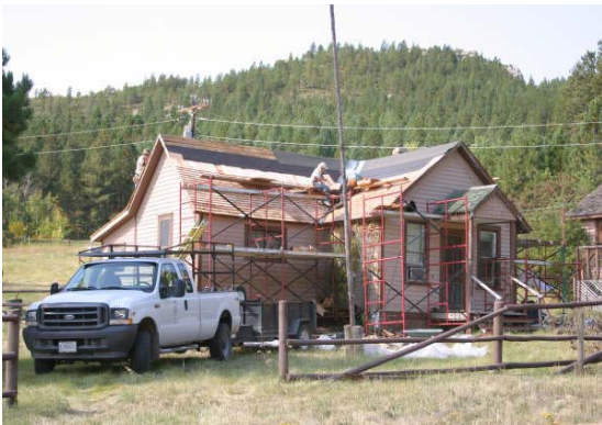
The R1 Team installing the new roof
