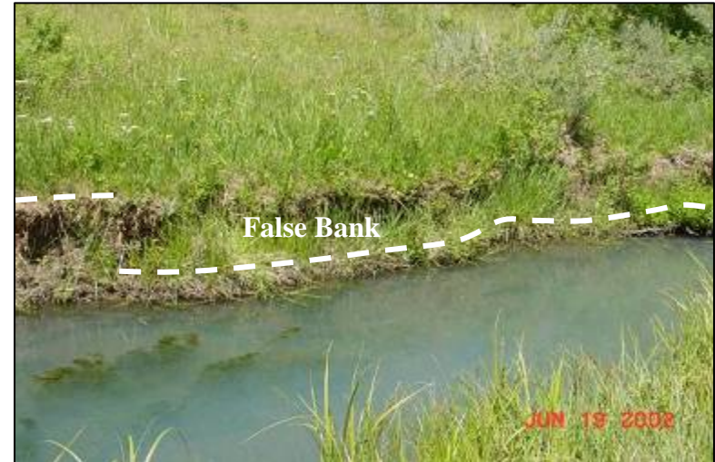
Figure 9 —false banks (FB) are reattached slump features covered with deep-rooted vegetation. They are an indicator of recovery and are considered stable.
