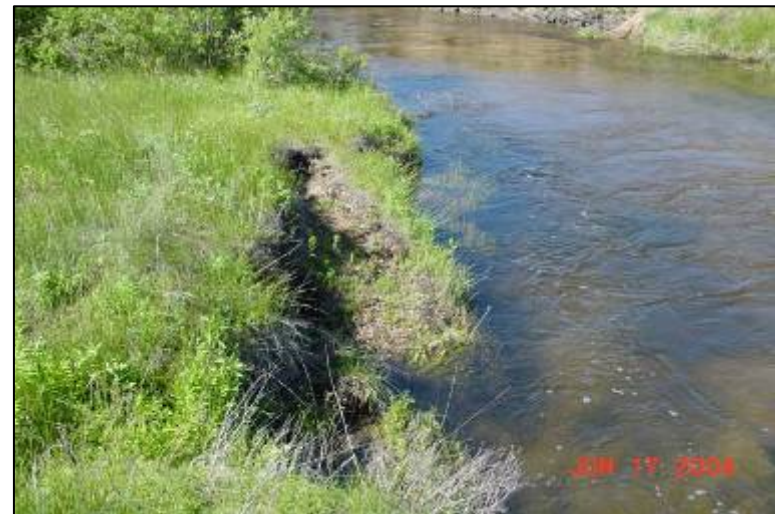
Figure 5 —the photo above shows a fracture and a large slump that is still attached to the streambank. Vegetation cover is at least 50 percent cover and is classified as covered/unstable (CU). (See Illustration 4.)
