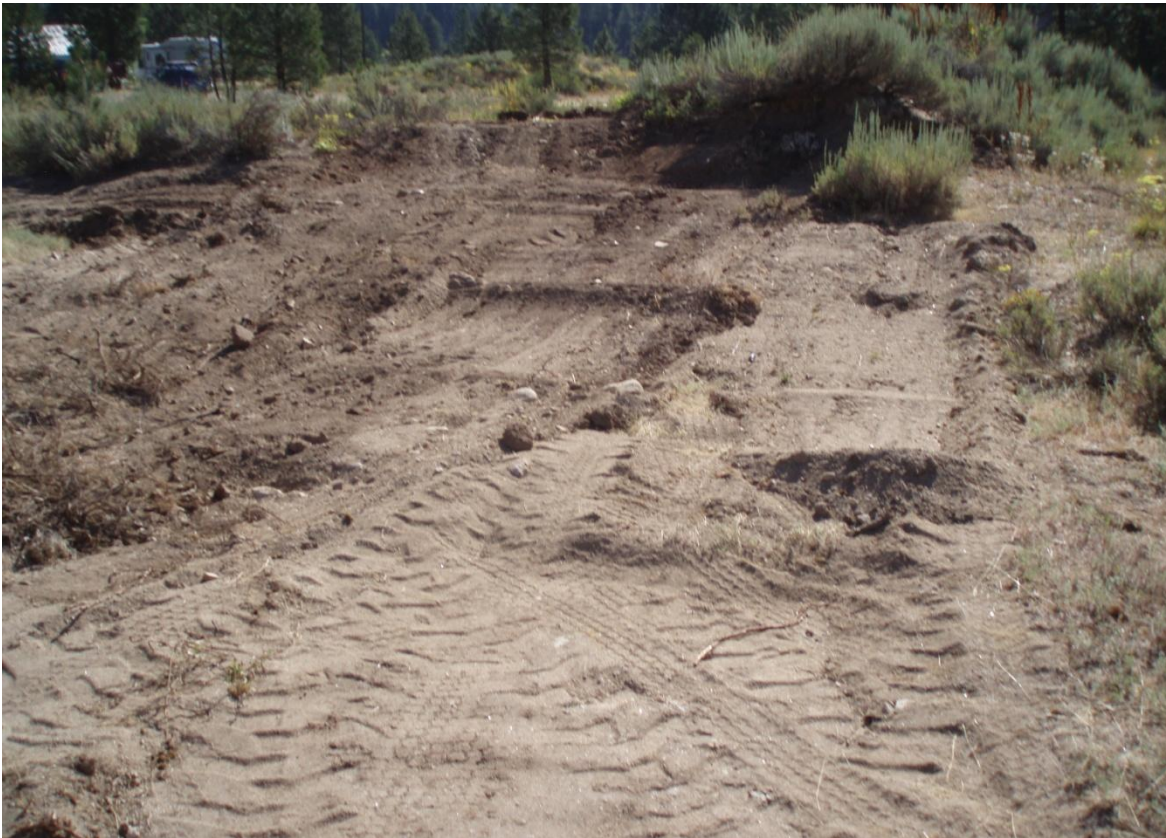
Photo 2 – A trenched area that was expanded to recover placer gold. The area has been re-sloped and is ready
