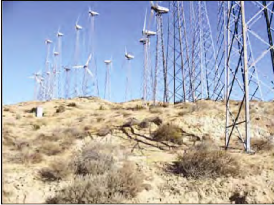
View of existing wind turbines and location of proposed wind turbine towers 18, 19, and 20.
