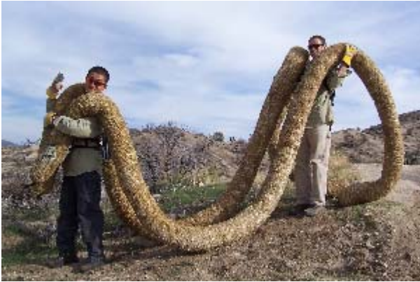
SCA crew carries large straw wattles for erosion control in Big Morongo ACEC.
