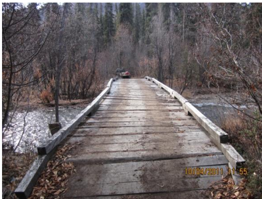
Bridge on Suslositna Creek trail
