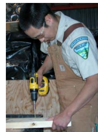
TOP PHOTO: The cabin crew on the porch of the new Foothills safety shelter between Shaktoolik and Unalakleet. RIGHT: Mike Prince of Emmonak is a Job Corps carpentry student who helped construct the new shelters.
