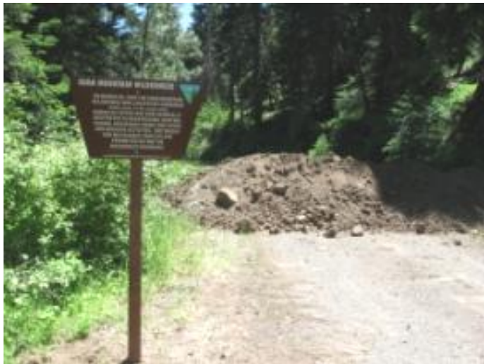
Earth berm barricade preventing vehicular access into the new Soda Mountain Wilderness.
