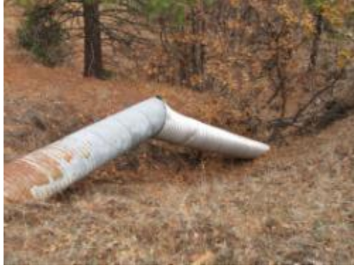
Culvert in the wilderness.
