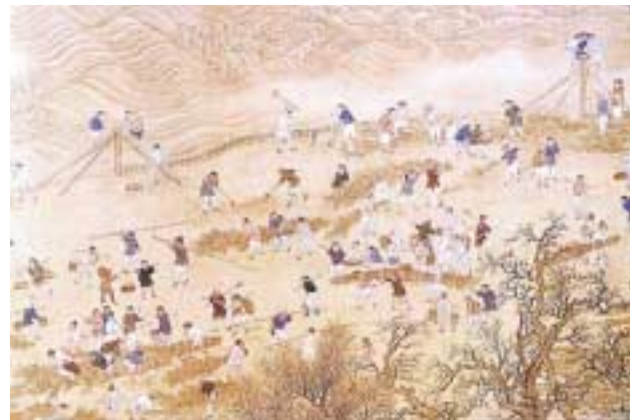
China 28 B.C. Bundling live stems for use in riverbank and dike repair. Kevin Finney
