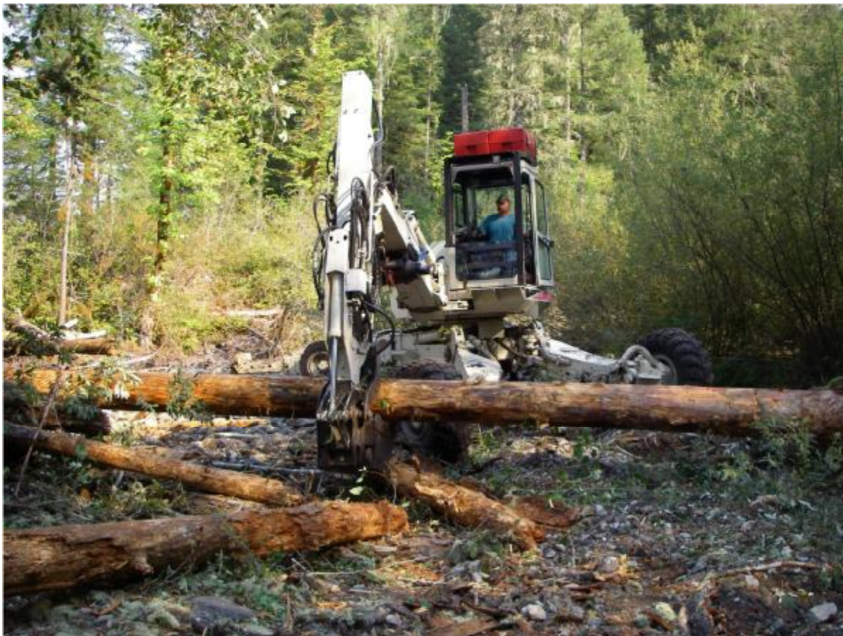
A Spyder excavator places logs in Elkhorn Creek.
